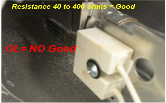
Igniter mounts on the Burner Ass'y
